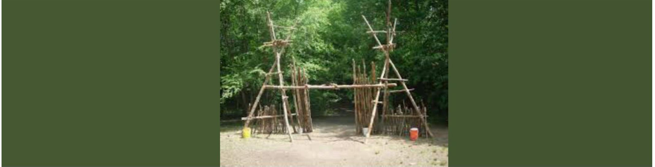
**Pioneering** is the art of using ropes and **wooden** spars **joined** by lashings and knots to create a structure. **Pioneering** can be used for constructing small items such as camp gadgets up to larger structures such as bridges and towers. These may be recreational, decorative, or functional.
